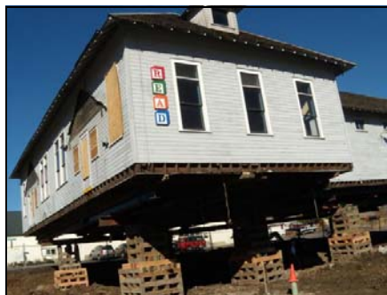
Raising the Building,
